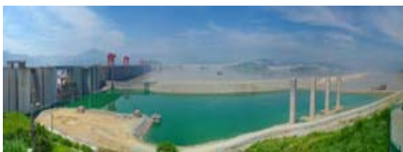
The upstream side of the Three Gorges Dam prior to filling the reservoir. Image courtesy of Wikipedia Commons
