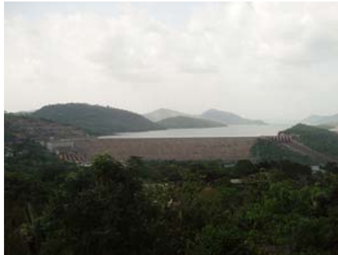
Akosombo Dam as seen from the Volta Hotel. The Akosombo Dam, built between 1961 and 1965, is 366 m. wide, 111 m. high, and 660 m. long. Its reservoir, Lake Volta, is the largest human made lake in the world. Public Domain Image
